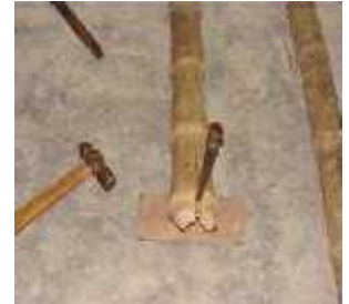
Fig.7 Half bamboo Splitting into three pieces.
