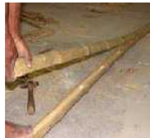
Fig.6 Bamboo splitting into Two pieces
