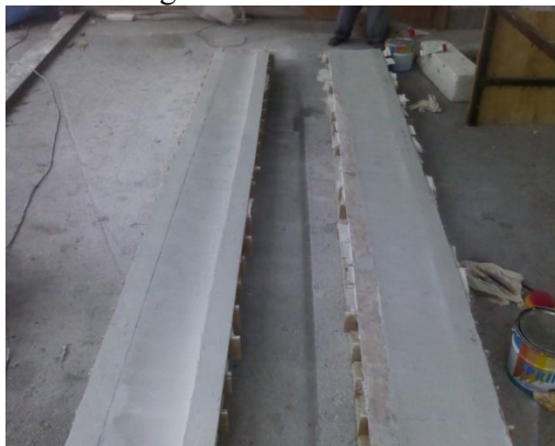
Step 11 Remove the cover sheet and smooth the surface using stucco
