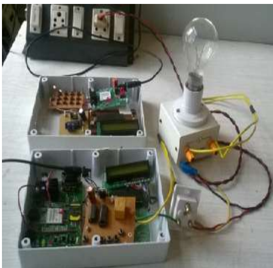
Fig3: Substation and Consumer Unit
