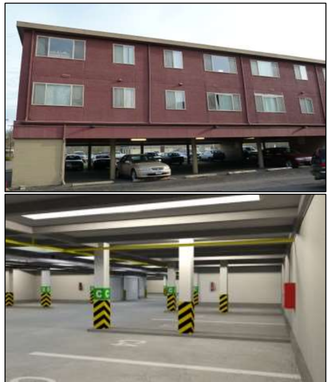
Fig 1: Building with soft-storey
