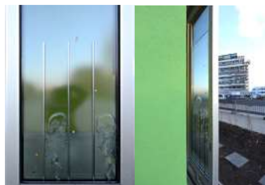
Fig.4- SolarLeaf – bioreactor façade
