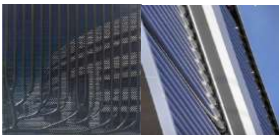
Fig.1- Glazing Integrated solar thermal façade collector
