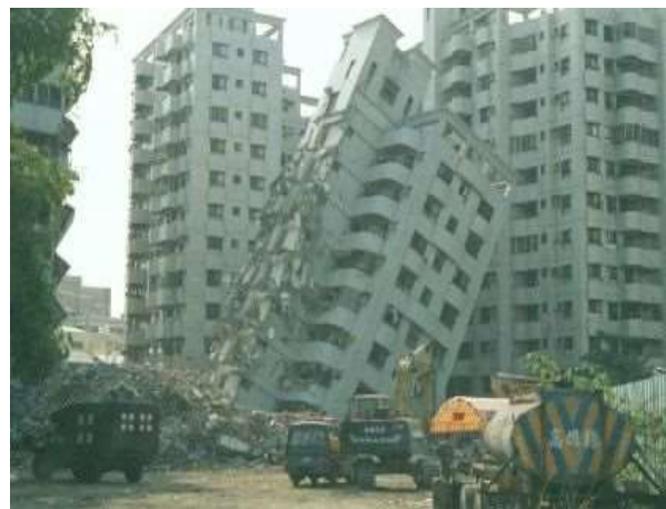
Fig. 1.2: Multi Storey Building affected by Earthquake at India
