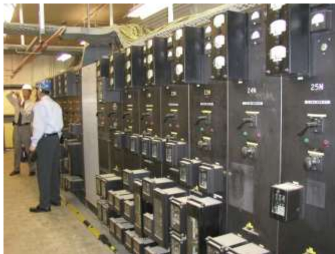
Fig. 5. Many discrete components lack the computing, memory, or communications capabilities required to be smart
